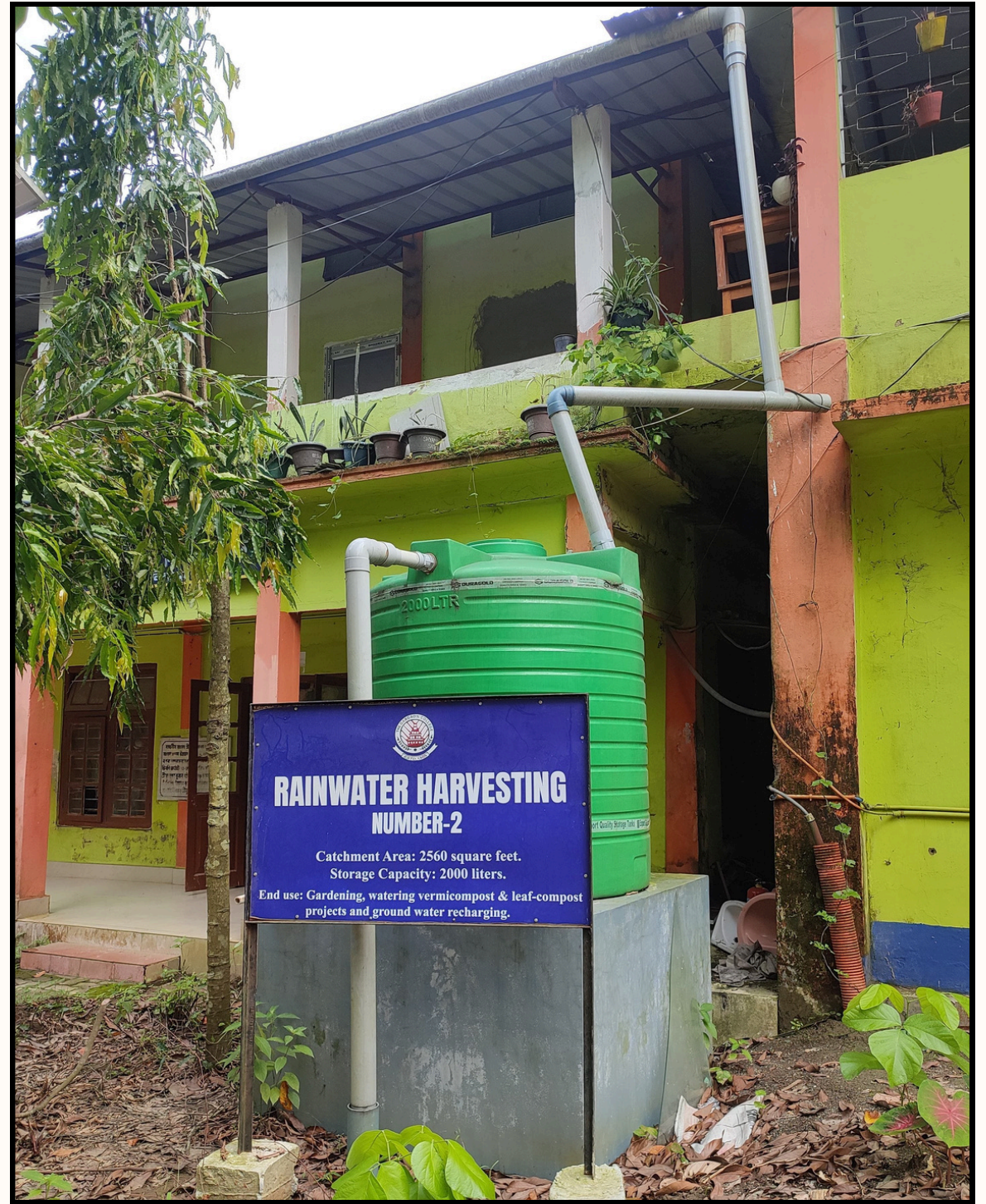
Rainwater harvesting tanks
