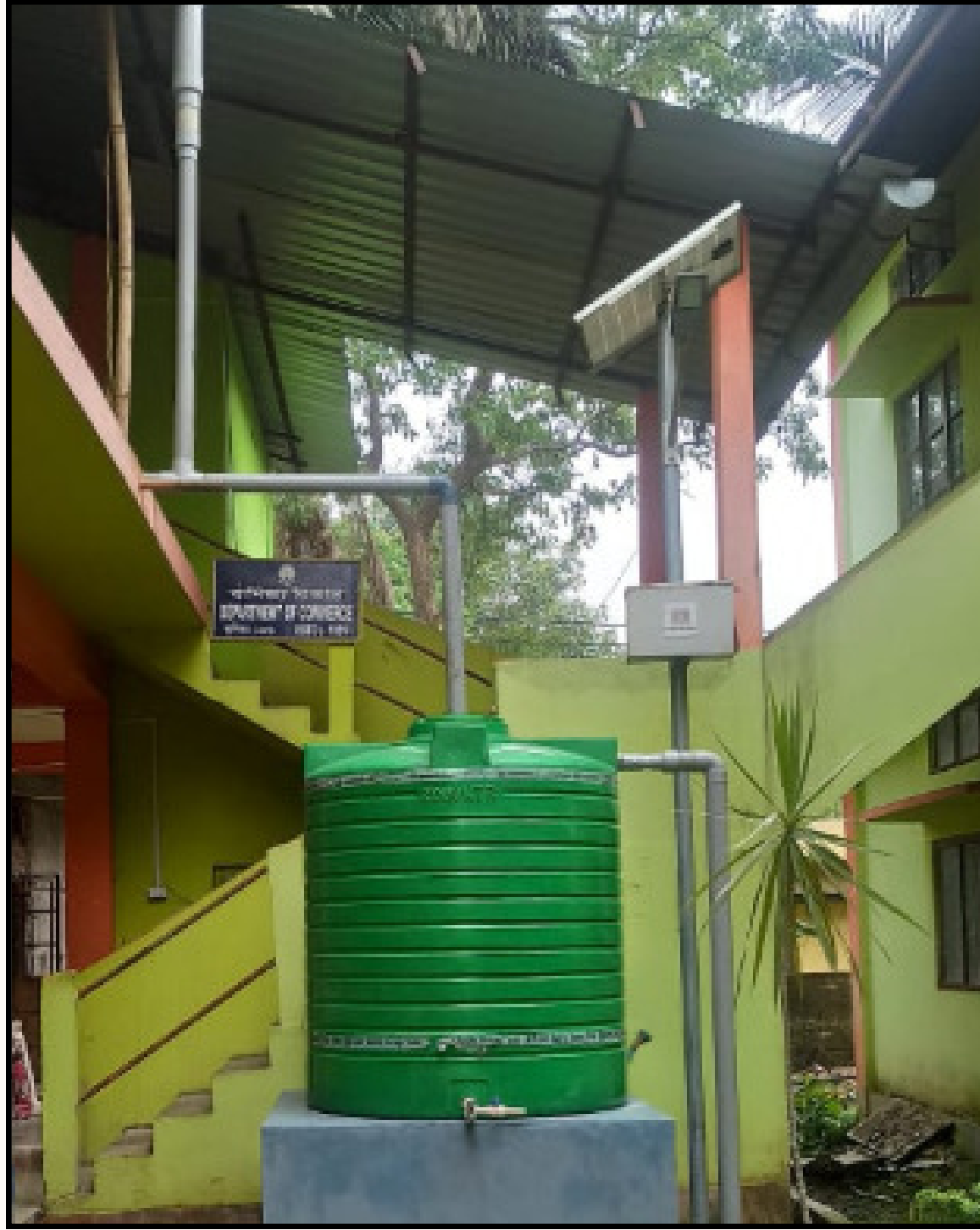
Rainwater harvesting tanks
