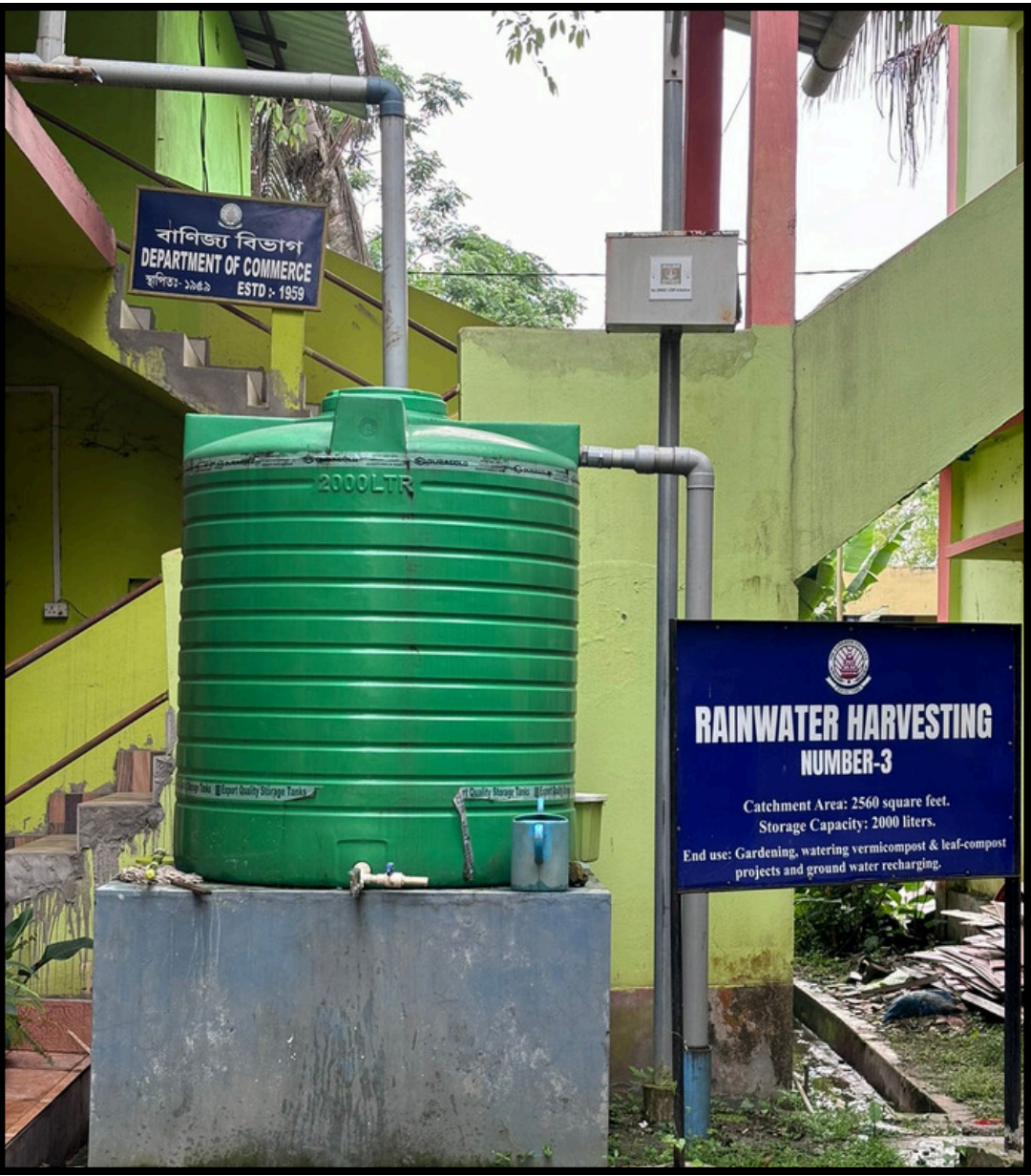
Rain water harvesting unit
